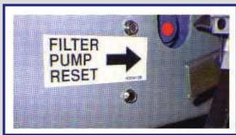
An overheated filter pump can be reset after it cools.
