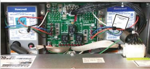
Relays are accessible on the interface board, behind the computer.
